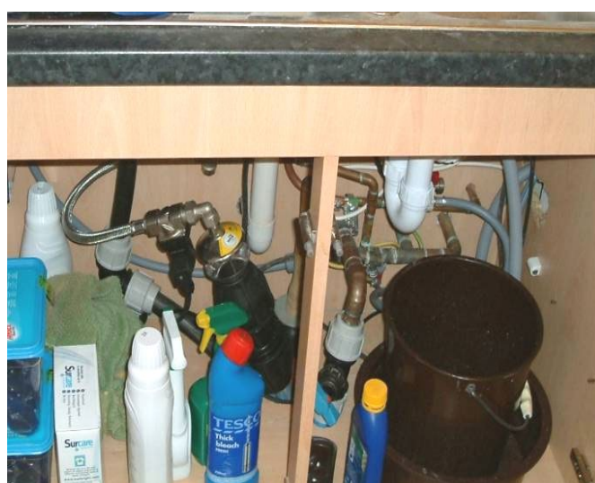
Example of poor installation, with no marking to clearly identify rainwater from mains water.
