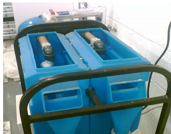
Internal back-up supply module with twin supplies and Type AB air gaps.
