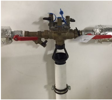
Fig 10: reduced pressure zone (RPZ) valve
