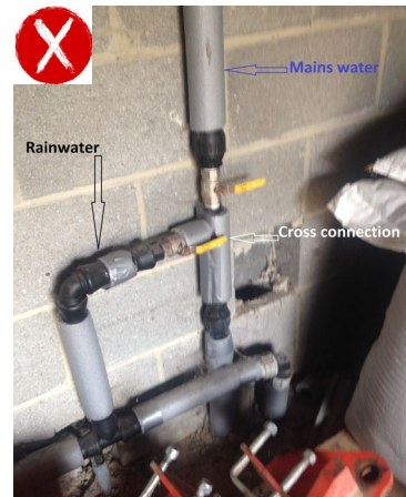
Fig 16: example of a cross connection between a rainwater and drinking water system
