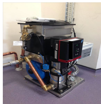
Fig 2: Storage cistern (break tank) supplying school laboratory
