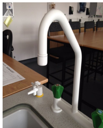
Figure 6: non concussive hose union taps (sometimes called hoseless taps) must be fitted in Fig 3: Scenario B – rooms 2, 3, &4. The tap gap must be maintained at all times
