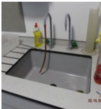
Figure 5: hose union taps are only permitted when backflow protection is in place (e.g. supplied from a storage cistern). The hose compromises the tap gap.
